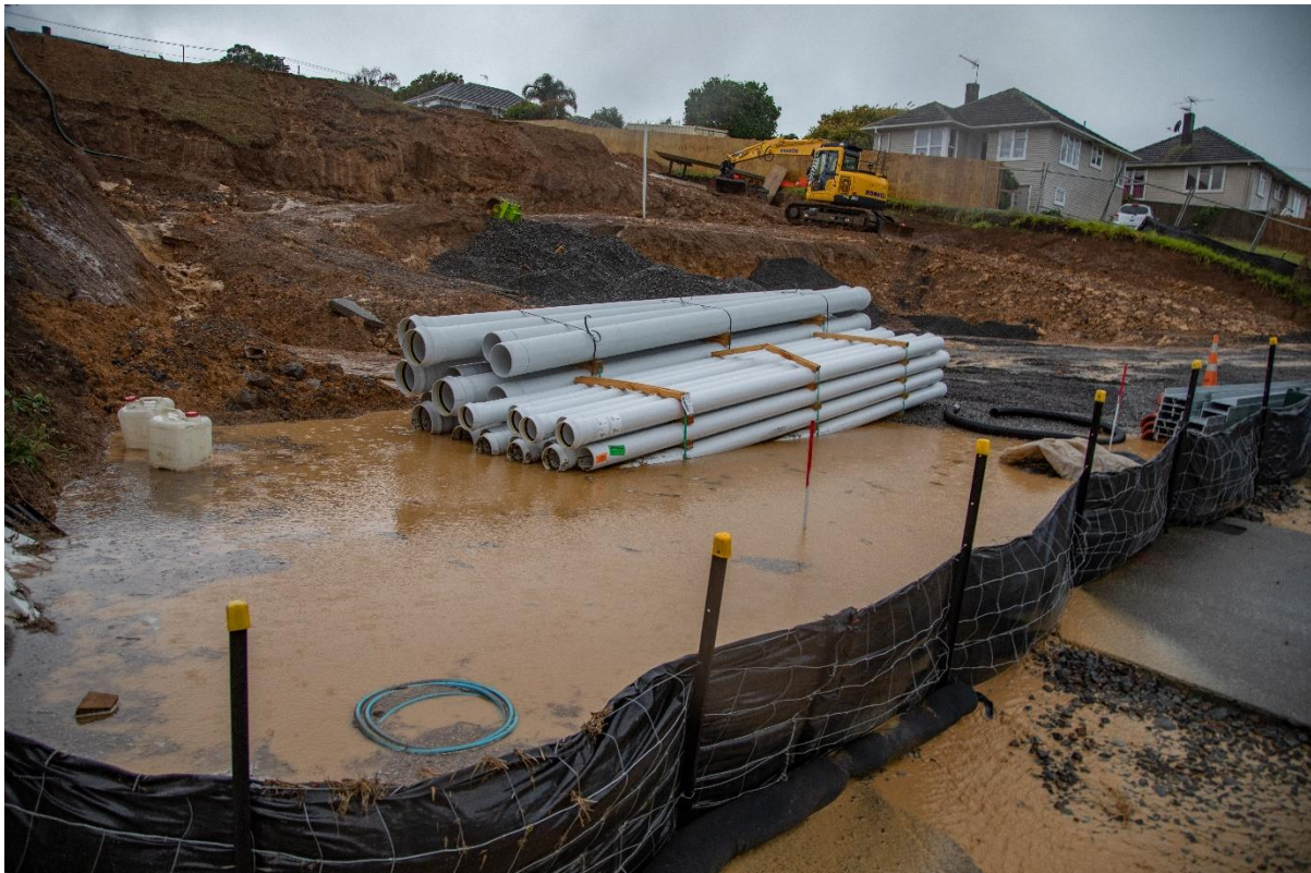
Building site in Glen Innes. Photo Shaun Lee
